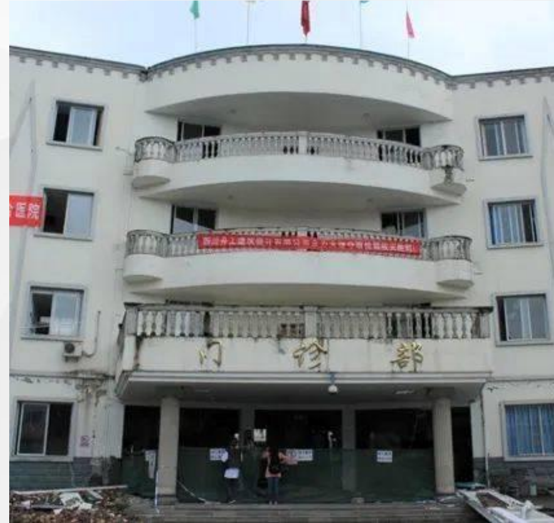
Traditional earthquake-resistant Old Outpatient Building of Lushan County People's Hospital
