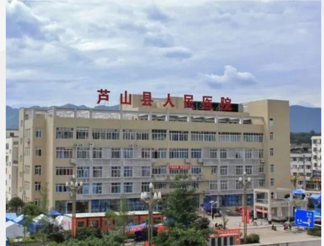
New Outpatient Building of Lushan County People's Hospital
