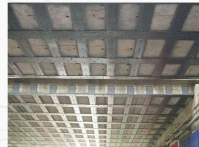
Bonded steel plate reinforcement for cast-in-place slab
