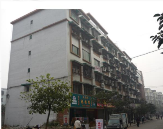
A residential building after the 2008 Wenchuan earthquake
