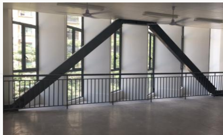
Bracing reinforcement method with Buckling-Restrained Braces (BRBs)
