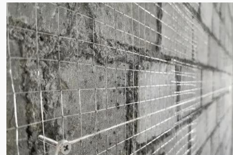
Masonry wall reinforcement method using high-toughness fiber-reinforced concrete overlays
