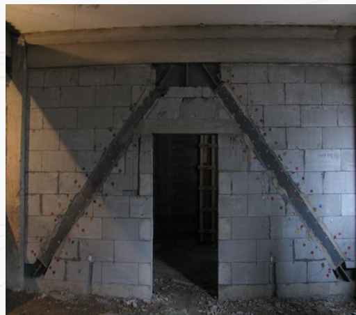
Support reinforcement node
