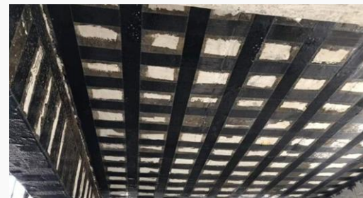
Bonded fiber cloth reinforcement for cast-in-place slab
