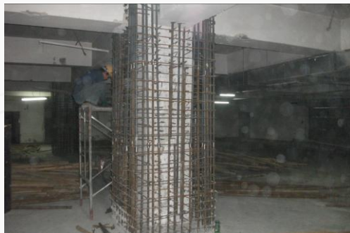
Section enlargement strengthening method for frame columns
