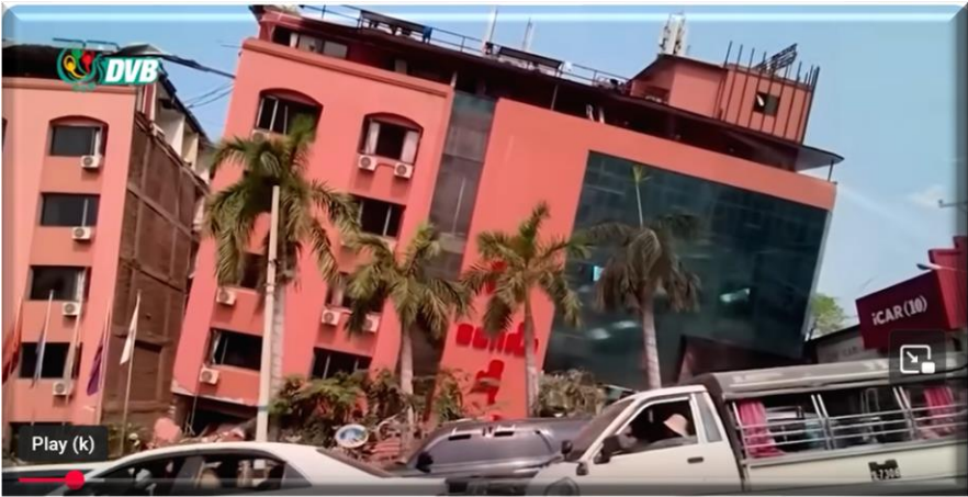
Foundation Soil Failure
