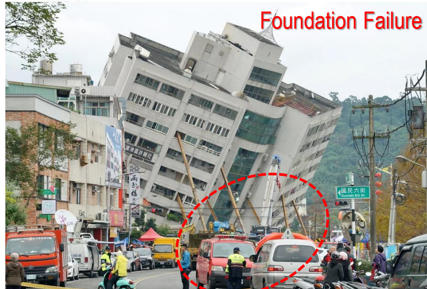
Rescue workers block off the area outside a building that tilted to one side after its foundation collapsed in Hualien, Taiwan.
