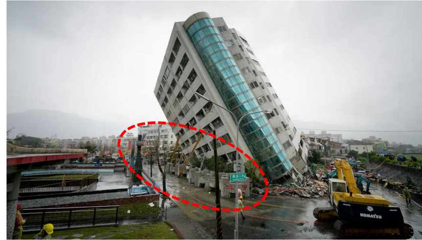
Rescue workers block off the area outside a building that tilted to one side after its foundation collapsed in Hualien, Taiwan.
