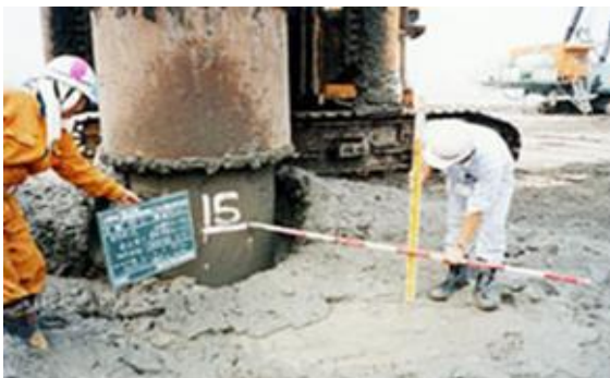
Figure 5.3-23 Measurement of Drill Core Position
