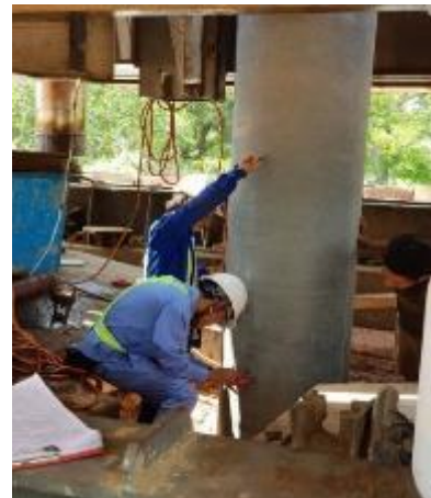
Figure 7.3-24 Measuring for Inclination
