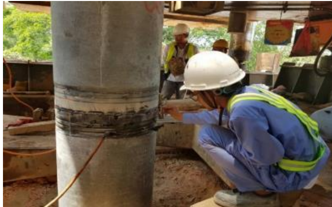
Figure 7.3-27 Welding Work Condition
