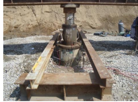
Figure 5.3-2 View of Static Loading Test
