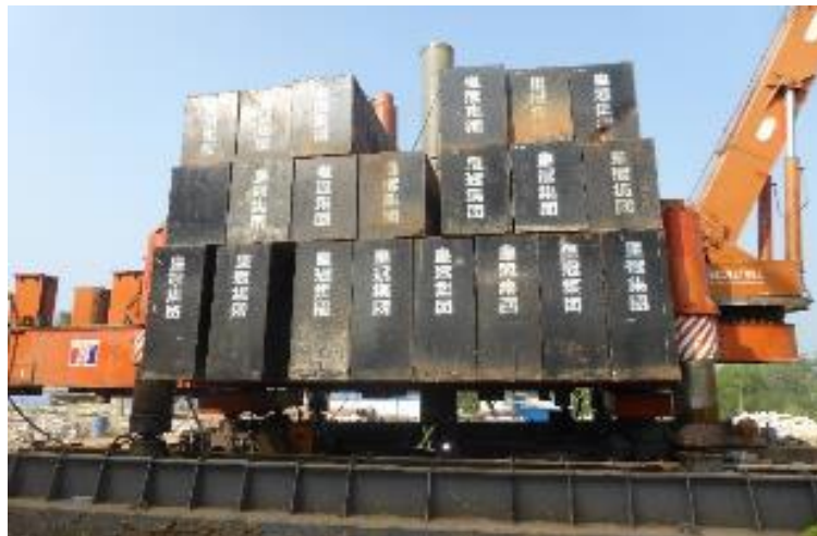
Figure 7.3-1 Basic Procedure of Jack in Piling Method
