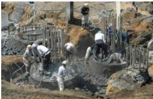
Figure 6.1-31 Pile Head Treatment
