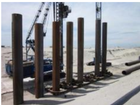
Figure 1.2-6 Steel Pile Construction
