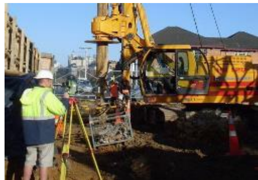
Figure 5.3-24 Survey for Drill
