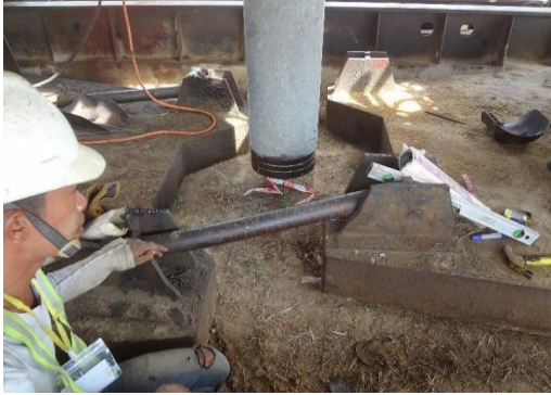
Figure 7.3-21 Centering of the Pile to Designed Point
