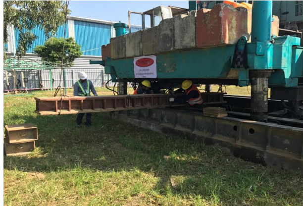
Figure 7.3-31 Preparation of Main Beam onto Machine Body
