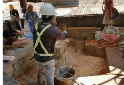
Figure 7.3-22 Measuring for Alignment
