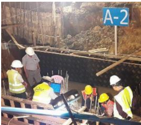
Figure 5.3-27 Sonic Integrity Test by MOC Engineers
