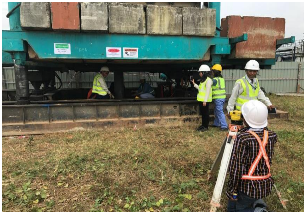
Figure 7.3-23 Measuring for Elevation
