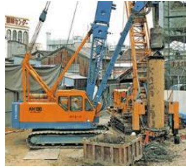
Figure 6.1-3 Shaking Excavator
