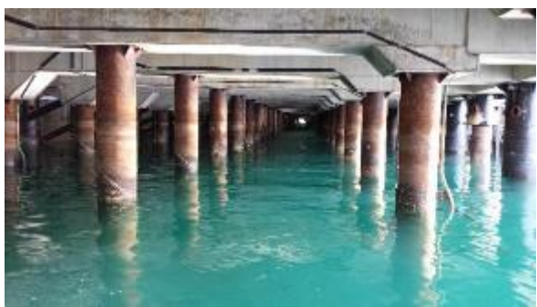
Figure 1.2-7 Steel Pile on River
