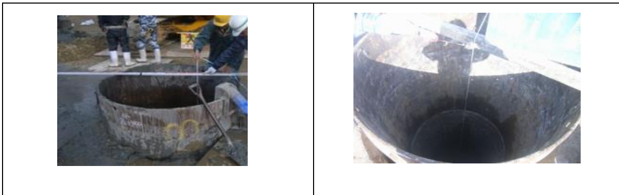
Figure 6.2-21 Measurement of Slurry Sediment
