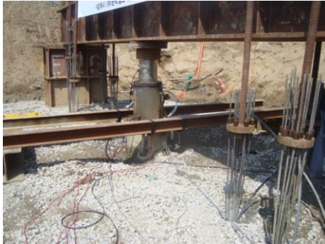
Figure 5.3-1 View of Static Loading Test
