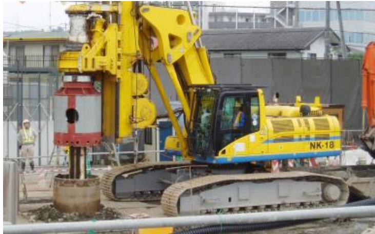
Figure 6.2-3 Excavation Machine for Earth Drilling Method
