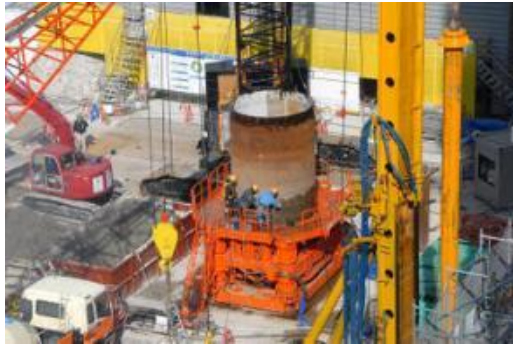
Figure 6.1-2 Rotary Excavator
