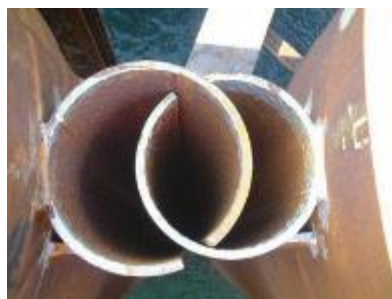
Figure 7.4-3 Joint of Steel Pipe Sheet Pile
