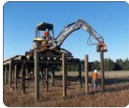
Figure 1.2-3 Timber Pile Construction
