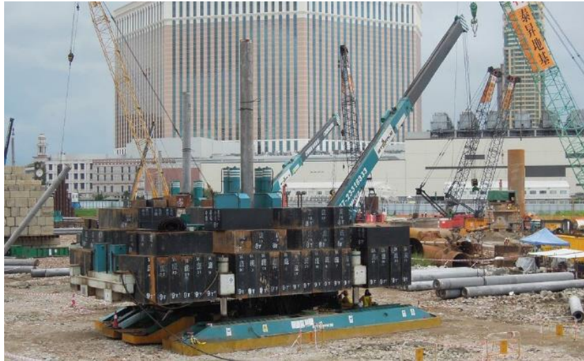
Figure 7.3-15 Pressing Driver
