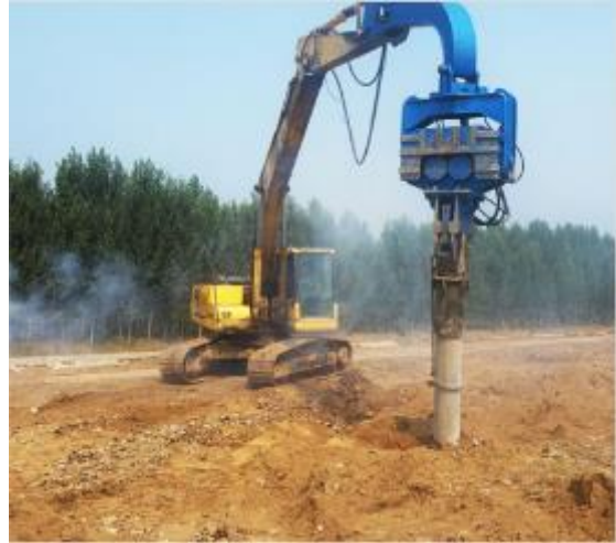
Figure 7.1-6 Vibratory Hammer:
