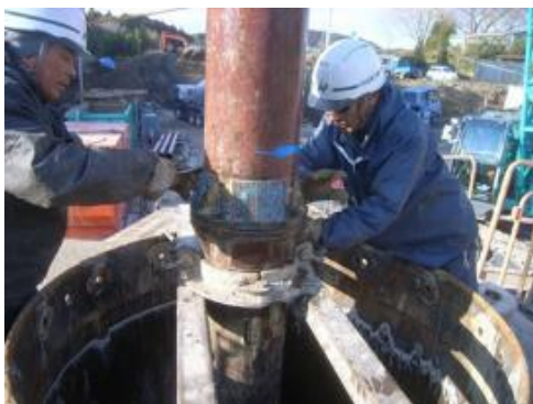
Figure 6.1-25 Flange Type Tremie Pipe
