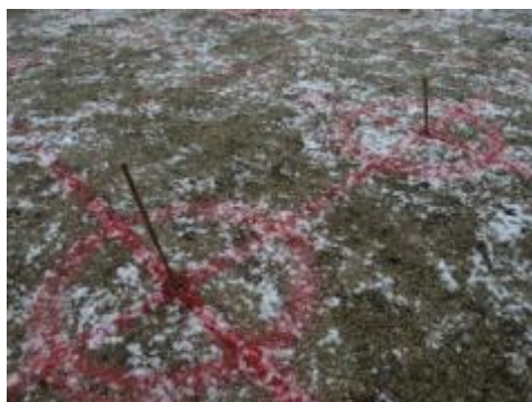
Figure 7.1-11 Pile Center Position
