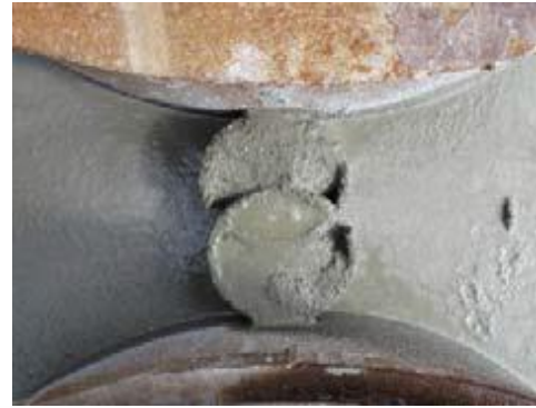
Figure 7.4-14 Joint Filled by Mortal
