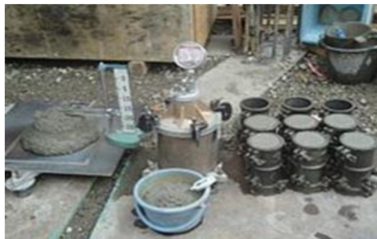
Figure 5.3-22 Testing Concrete on Site
