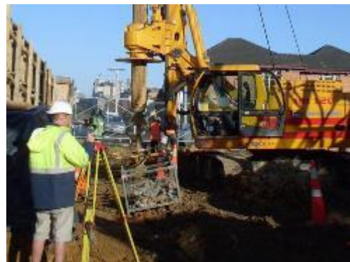
Figure 7.2-8 Survey of Drill Core Position
