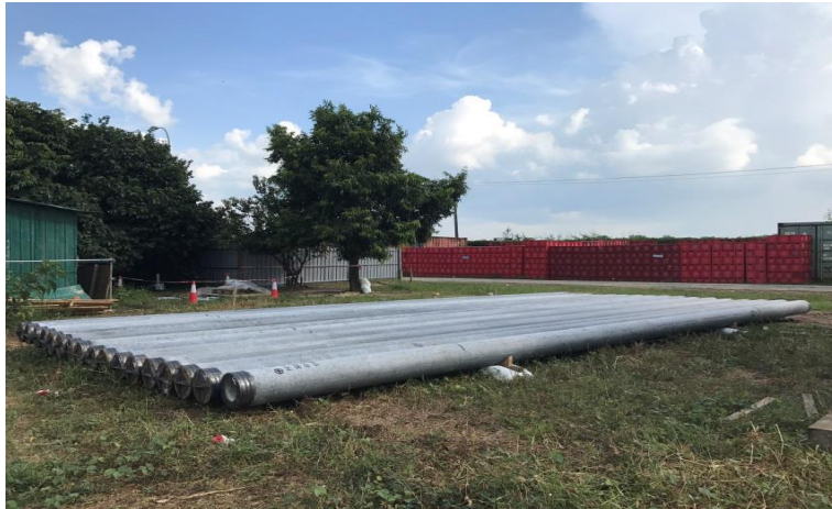
Figure 7.3-14 Storage Condition of Pre-stressed Spun Pile Product
