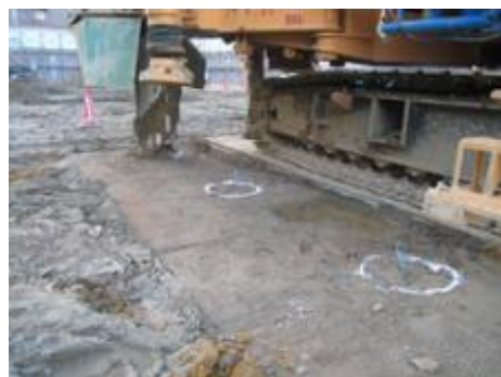
Figure 7.1-11 Pile Center Position
