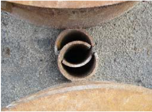
Figure 7.4-14 Joint Filled by Mortal
