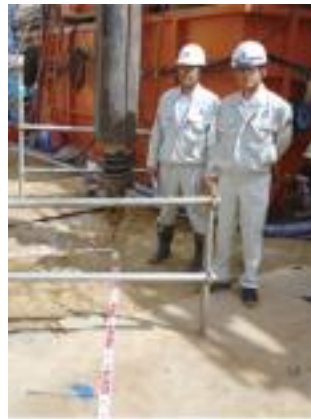
Figure 7.2-7 Measurement of Drill Core Position
