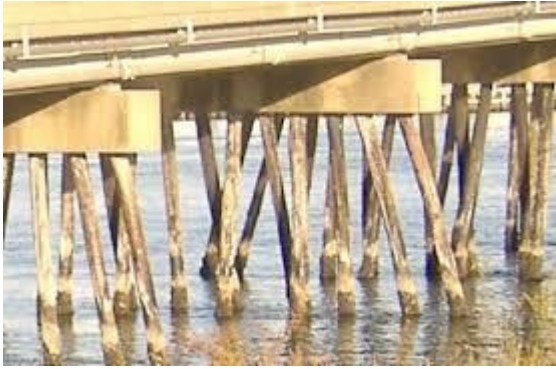
Figure 1.2-2 Timber Pile Foundation
