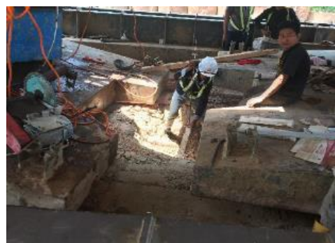
Figure 7.3-20 Measuring for Alignment
