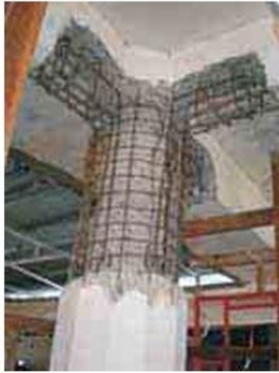
ADDITION OF STIRRUPS & ANCHORING
