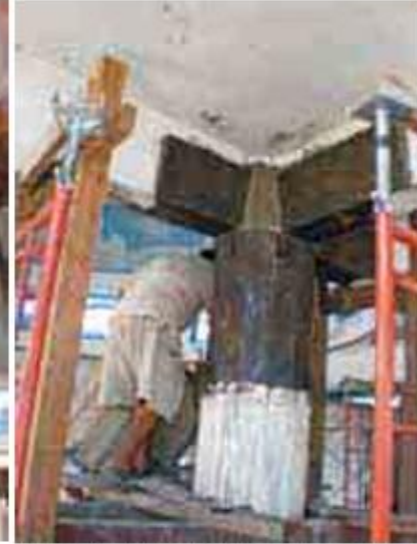
FORMWORK REMOVED AFTER CONCRETING
